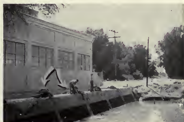
INHIBITING ALGAE IN ARIZONA (at left) by large-sized spray loaded with Rada. Below, masses of moss (see arrows) at Yuma's Boundary Pumping Plant being pulled up by weed hooks, before Rada made the job easier. Photos by the author.
